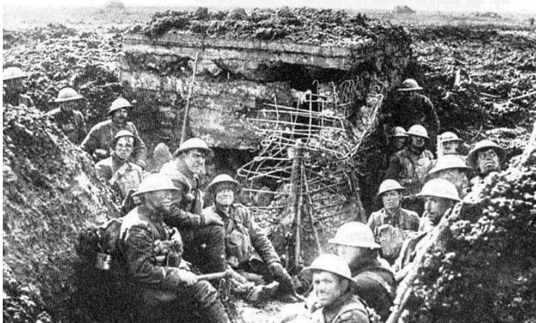
George Metcalf Archival Collection, Canadian War Museum A German machine-gun emplacement of reinforced concrete on the crest of Vimy Ridge, and the Canadians who seized it.
